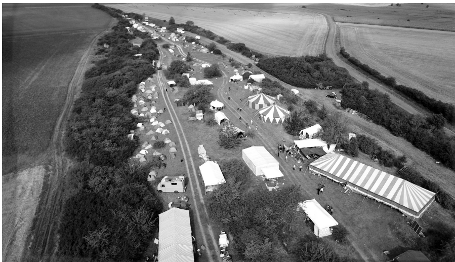
La Gare (the old Luméville station) during the Rayonnantes camp in 2021
